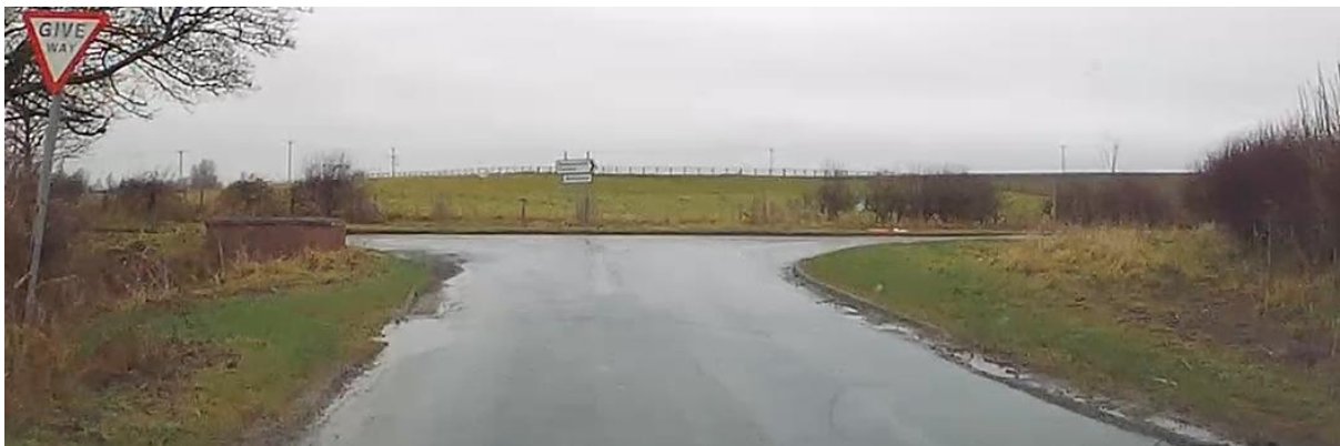
R2.22 - Condition score 0. (For Junction markings)
