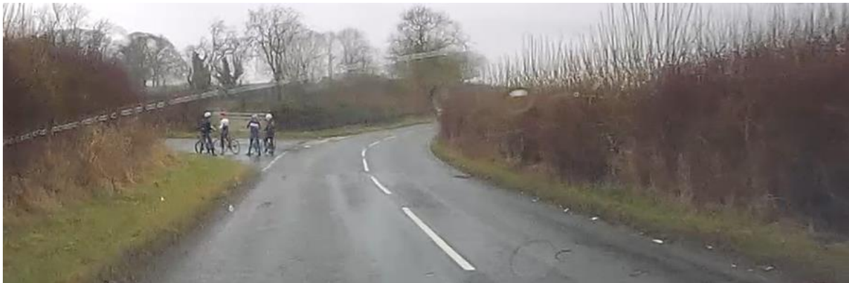
R5.23a - Condition Score 40 (Junction markings)
