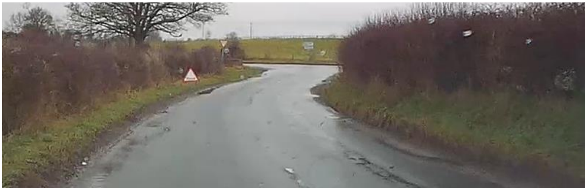
R2.22 - Condition score 0. (no markings approaching Junction)
