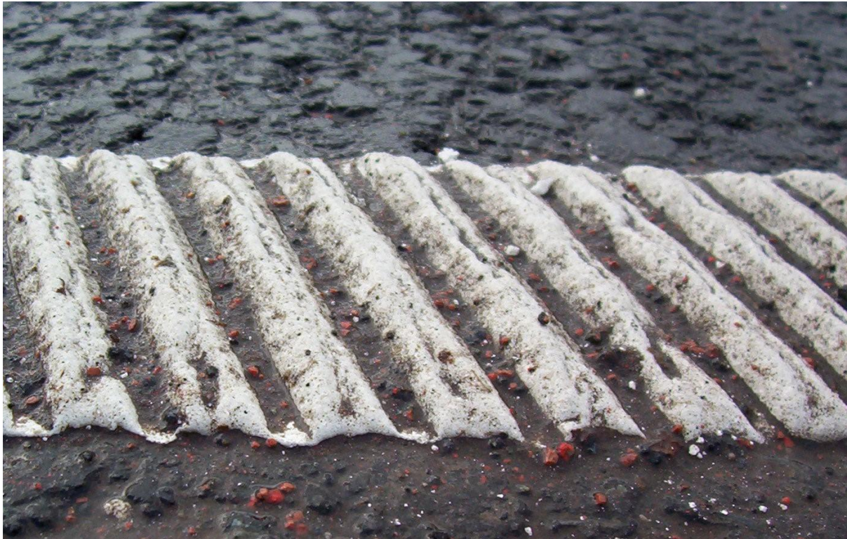
Figure C.3 Condition score 50 – long view
