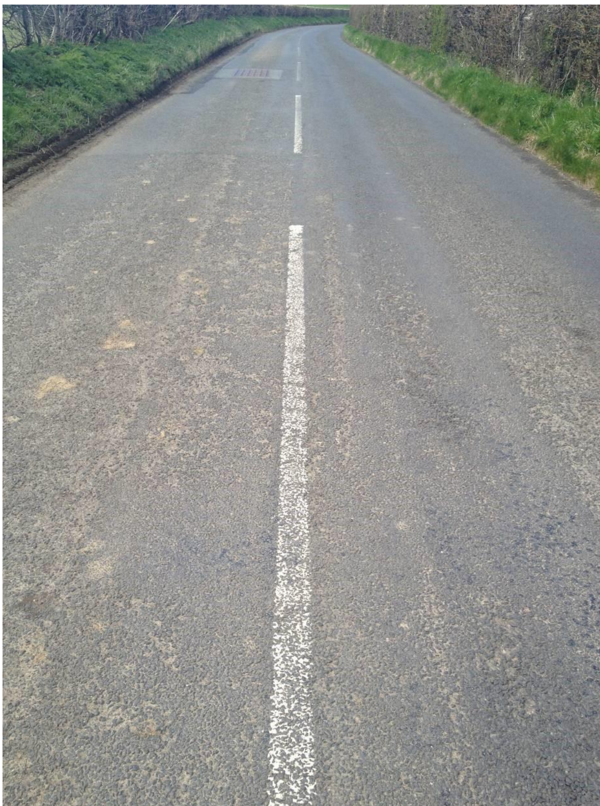
Figure C.12 Condition score 10 – long view
